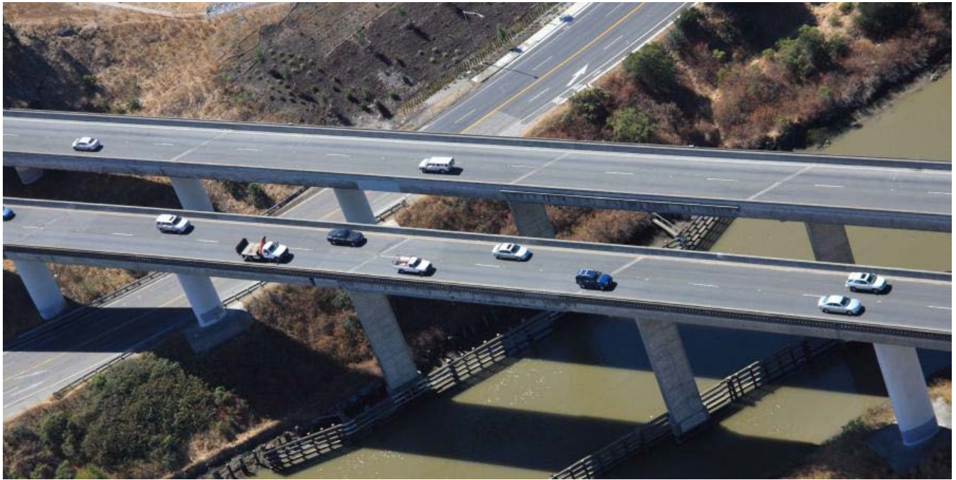
Figure 1: Difficult access to bridge-underside areas 75 feet above the Petaluma River
