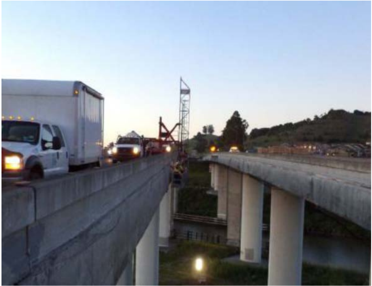
Figure 3: Difficult access to bridge columns during night-time lane closures
